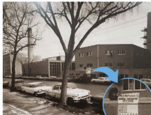
1960's Hospital Addition with Mortenson project signage
